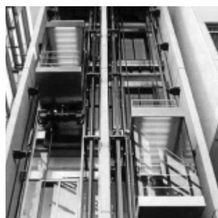
ELEVATOR & COMPONENTS CONSTRUCTION
